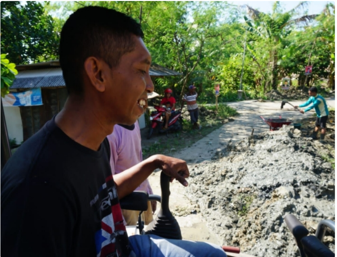
Sertu Abdul Aziz Sang Operator Excavator
